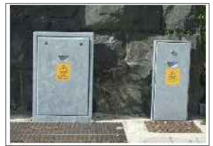
Image of ESB mini pillar with adjacent Public lighting micro pillar.
